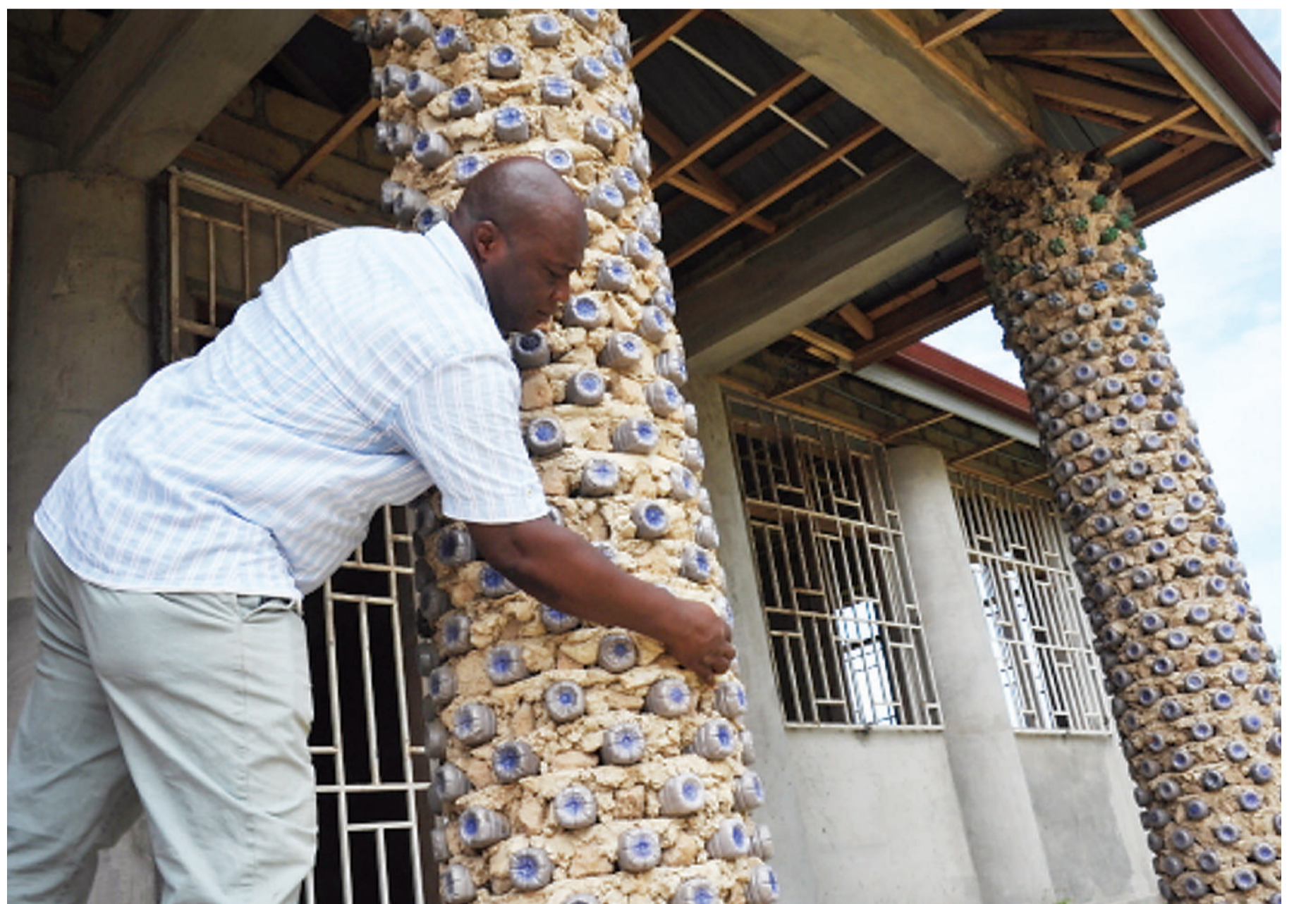
Zhoungbogbo shows recycled plastic bottles filled with soil, which are used as bricks for building a community library, in Accra, Ghana, on June 24, 2021. File photo
