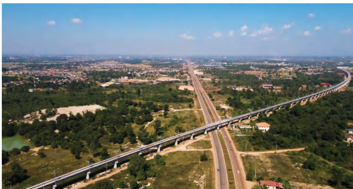
Aerial photo taken on Nov. 21, 2021 shows a section of the China-Laos Railway on the outskirts of Vientiane, Laos. Xinhua
