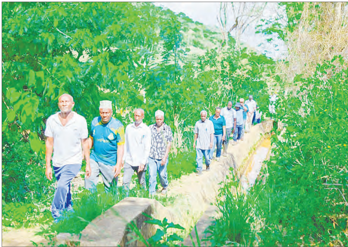
Farmers and experts from the National Irrigation Commission (NIRC) at Tubugwe Juu Irrigation Scheme in Kongwa District, Dodoma Region, during a visit to the infrastructure as part of training for Food Systems Resilience Project in Tanzania (TFSRP - P4R). Photo: Correspondent Renatha Msungu
