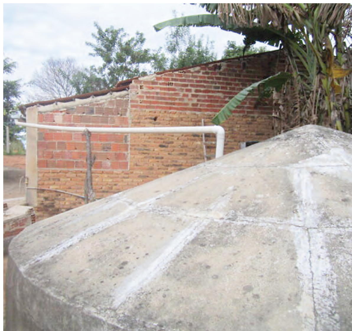
This 16,000-litre concrete slab tank stores rainwater collected on the roof and uses pipes to provide drinking water for Josaida Nunes and Eronildes Silva, in the Sertão de Pajeú, in Brazil's semiarid Northeast. CREDIT: Mario Osava / IPS
