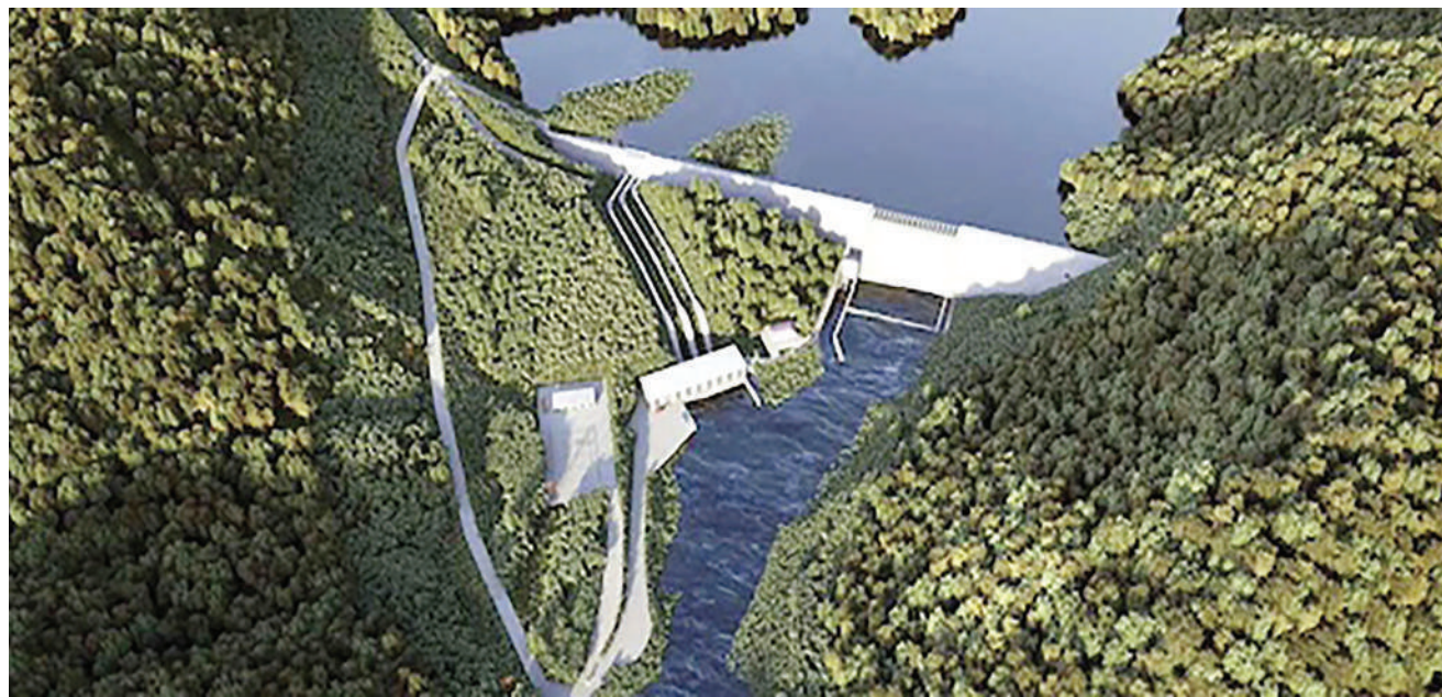
Hydropower plants like Kinguéé Aval in Gabon can, with refurbishment, play a key role in Africa's energy transition by reducing reliance on fossil fuel-derived electricity.
