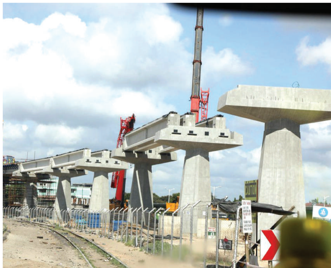
Construction work of the SGR infrastructure in Dar es Salaam.
