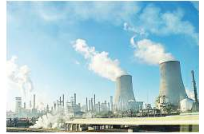
Sasol's synfuel plant in Secunda, Johannesburg.
