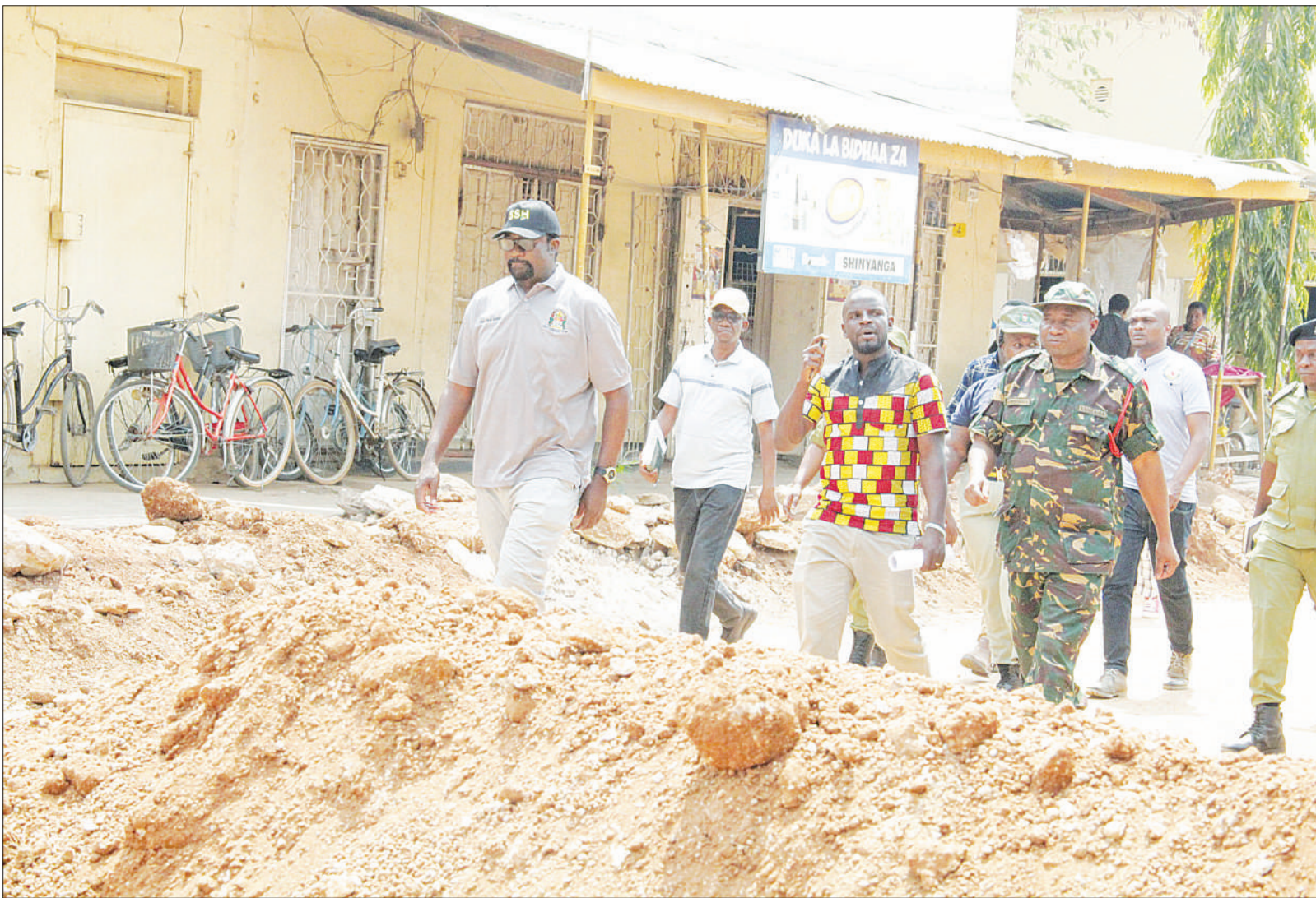
Shinyanga district commissioner Julius Mtatiro (L) makes an inspection tour of progress in the construction of roads and bridges yesterday. Photo: Correspondent Marco Maduhu
