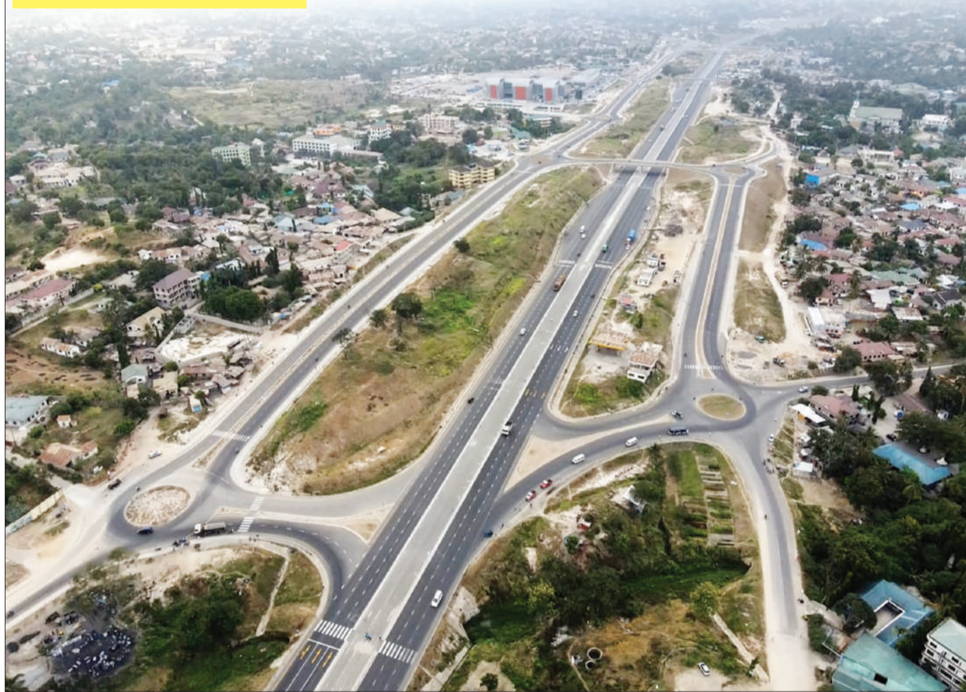
This is an aerial view of a section of the eight-lane Morogoro Road running from Kimara suburb in Dar es Salaam Region to Kibaha in Coast Region, as captured yesterday. Construction is reported to be 98 per cent done, with finishing touches expected to be completed by the end of next month. Photo courtesy of Works ministry
