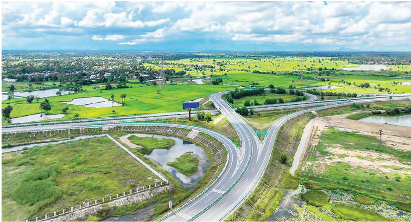
An aerial drone photo taken on Sept. 25, 2024 shows a section of the Phnom Penh-Sihanoukville Expressway in Kampong Speu province, Cambodia. (Cambodian PPSHV Expressway Co., Ltd./Handout via Xinhua)
