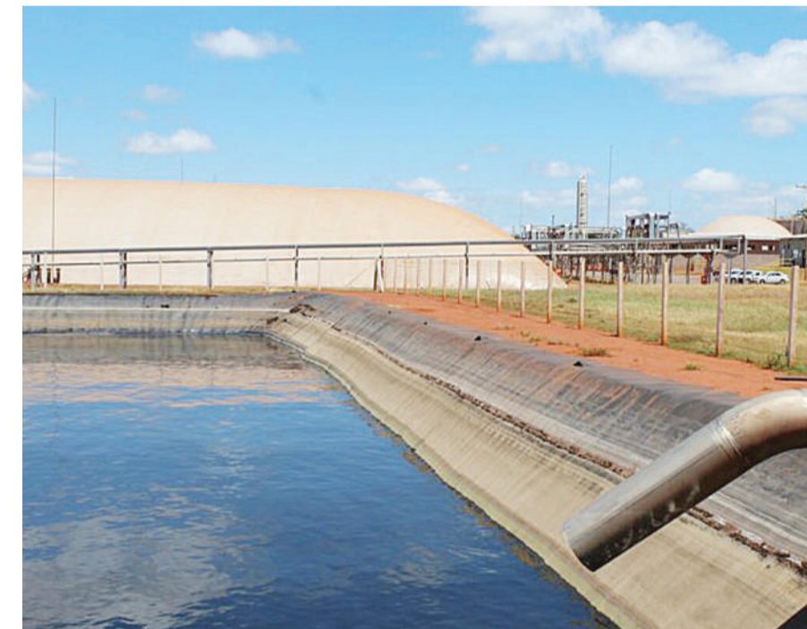
The vinasse pond at the Cocal plant, in the Brazilian municipality of Narandiba, feeds the biodigesters that produce biogas, later purified and refined for use in electricity generation or conversion into biomethane, a renewable and clean fuel equivalent to natural gas. CREDIT: Mario Osava/IPS
