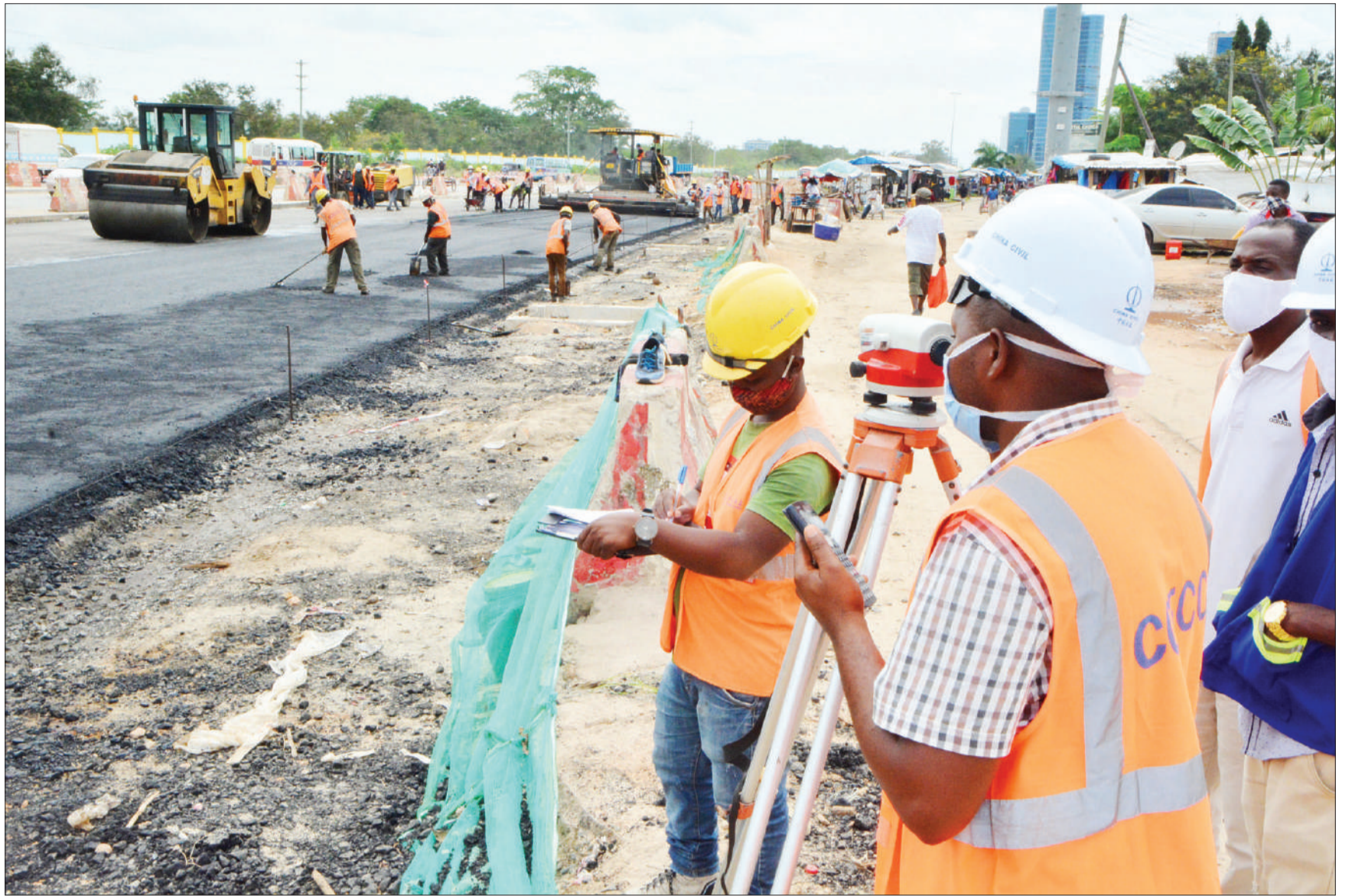
China Civil Engineering Construction Corporation site surveyors and other workers in business on Dar es Salaam's Sam Nujoma Road, as captured yesterday. Photo: Correspondent Miraji Msala
