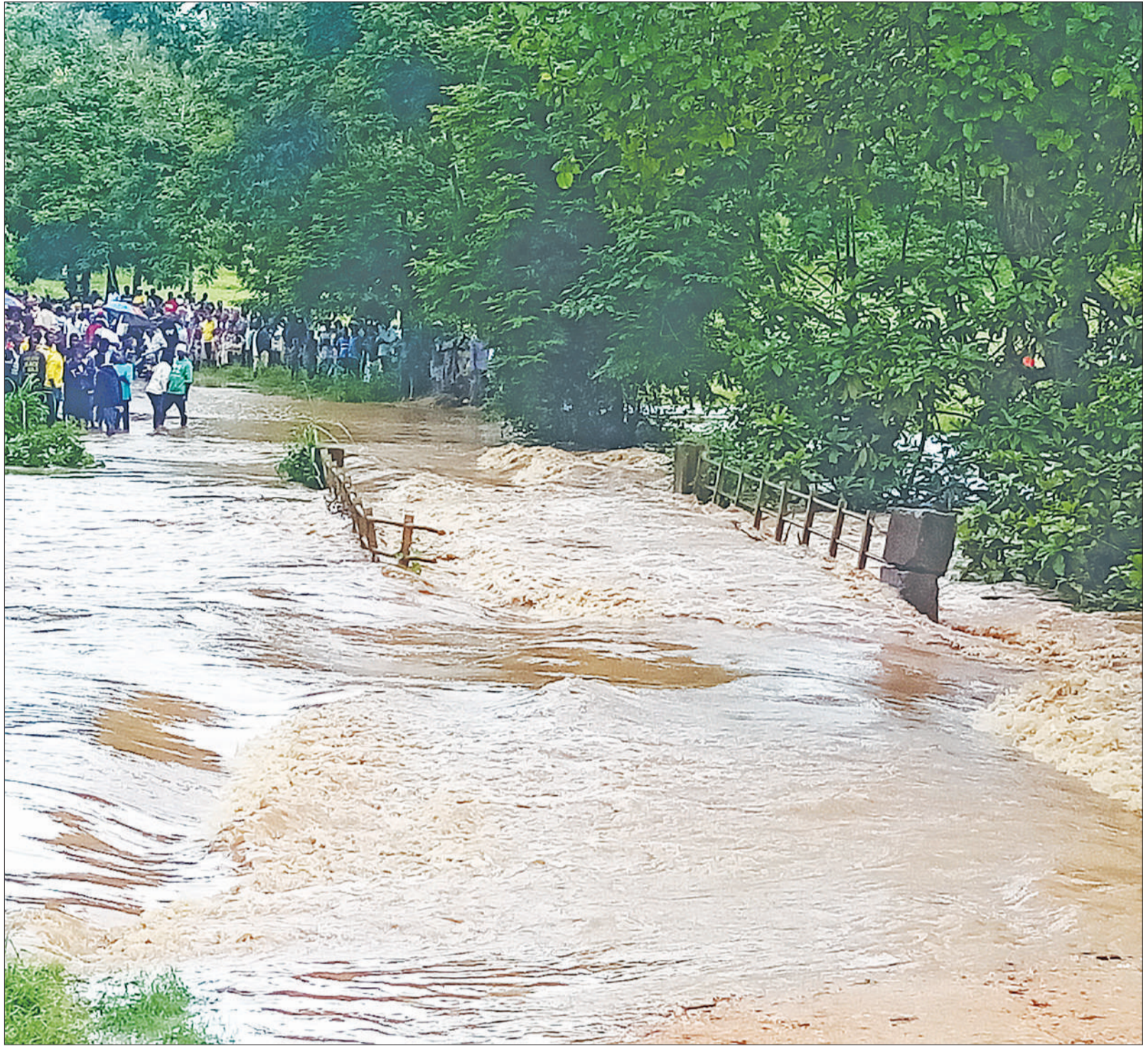
At least 200 people who were travelling by road between Muheza town and Kicheba and Misozwe villages in Amani ward stranded yesterday, with floodwaters having covered the strategic bridge pictured following the ongoing heavy rains. Photo: Guardian Correspondent
