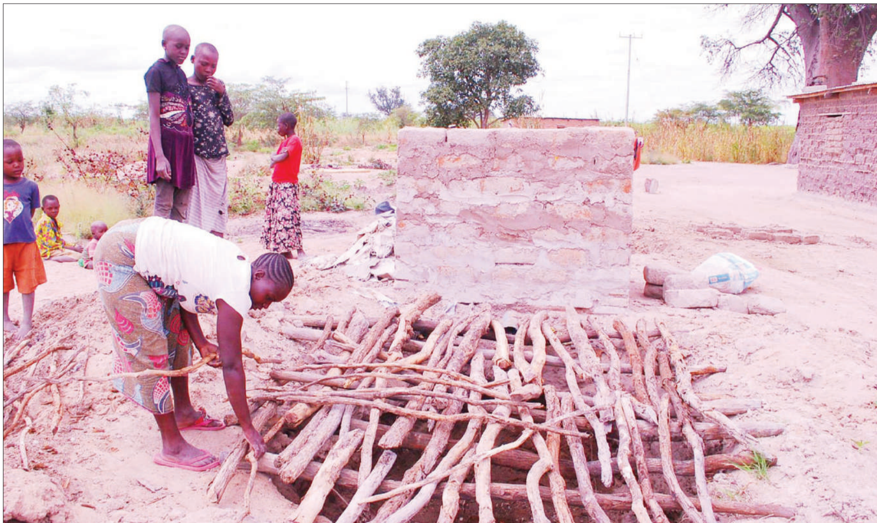
A resident of Bahi in Dodoma Region lays the groundwork for the construction of a pit latrine, as captured at the weekend. Photo: Correspondent Peter Mkwavila
