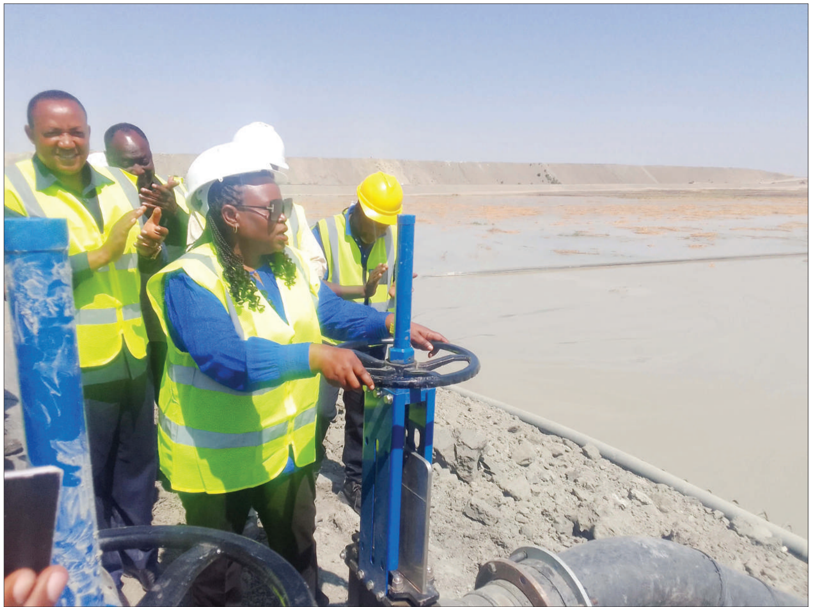
Shinyanga regional commissioner Christina Mndeme (in white helmet, foreground), symbolically operates a plant at the newly built mud dam at Mwaadui Mine yesterday to launch the resumption of diamond mining at the site. Activities ground to a halt after the dam previously in place burst on November 7, last year. Photo: Correspondent Marco Maduhu
