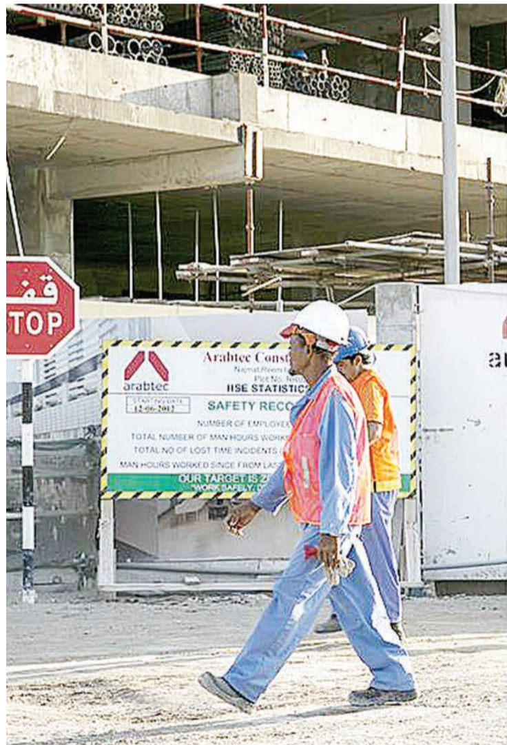
An Arabtec construction site in Dubai.
