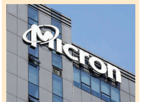
A Micron building. The US data storage producer is making a $15 billion investment in a fabrication site in Idaho, US. Photo: File
