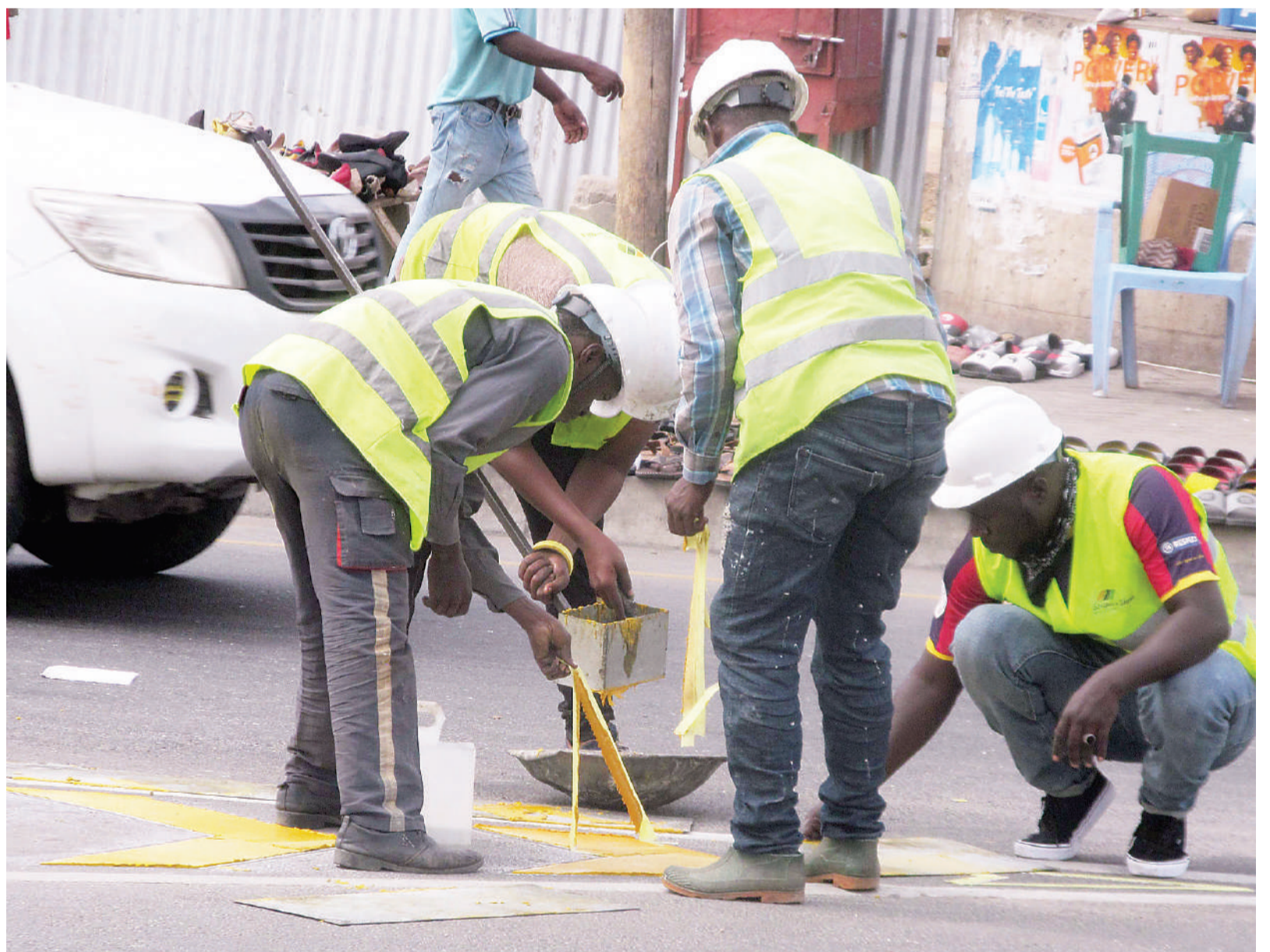
Painting of road signs well under way along a Mwenge section of Dar es Salaam's newly rehabilitated and expanded Bagamoyo Road, as found yesterday. Photo: Correspondent Sabato Kasika
