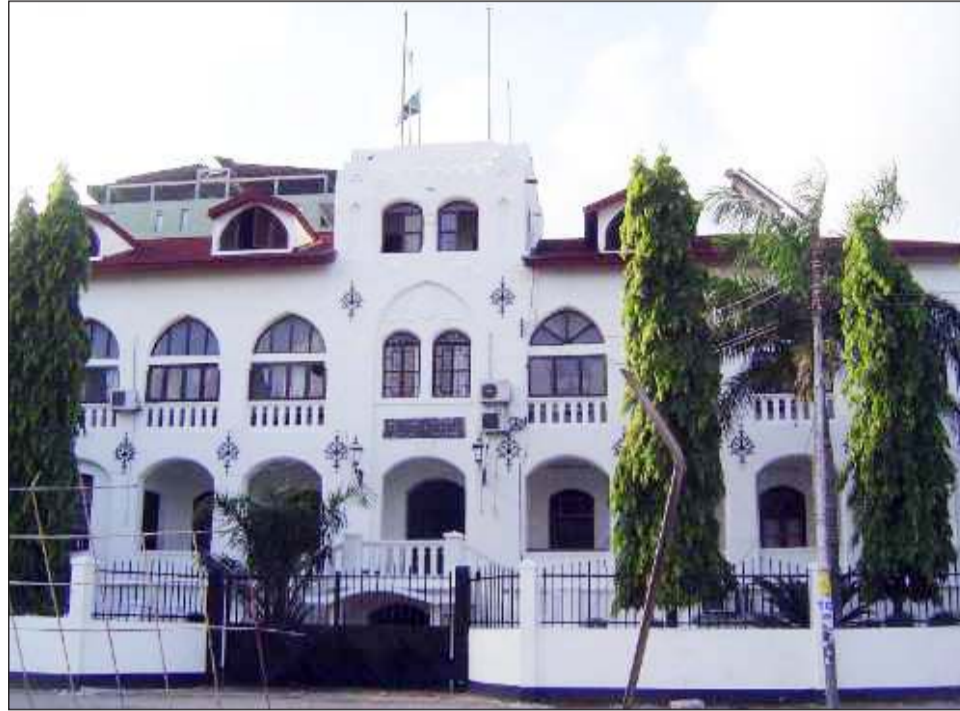
Dar es Salaam City Council offices on Samora Avenue. A beautiful restored old colonial building, which gives prestige to the area, and should be valued by those using it, and for passersby who enjoy seeing it. Such structures add character to places that lack architectural interest or history. (file photo)
