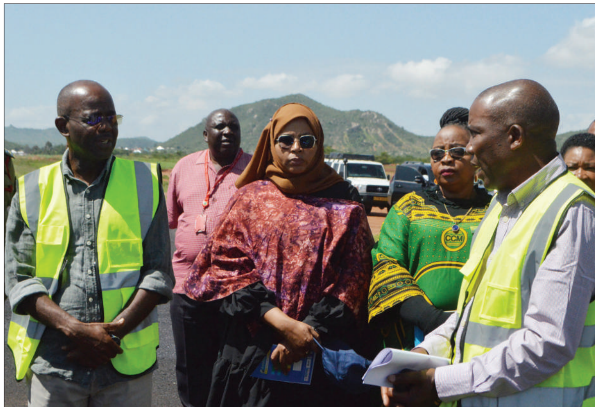
Daniel Kindole (R), Iringa regional manager of the Tanzania National Roads Agency (Tanroads), pictured in Iringa municipality yesterday briefing Works and Transport minister Prof Makame Mbarawa (L) on progress made in renovating and expanding Iringa Airport. He said the work was 45 per cent done. The minister was on a one-day tour of Iringa Region. Photo: Correspondent Friday Simbaya
