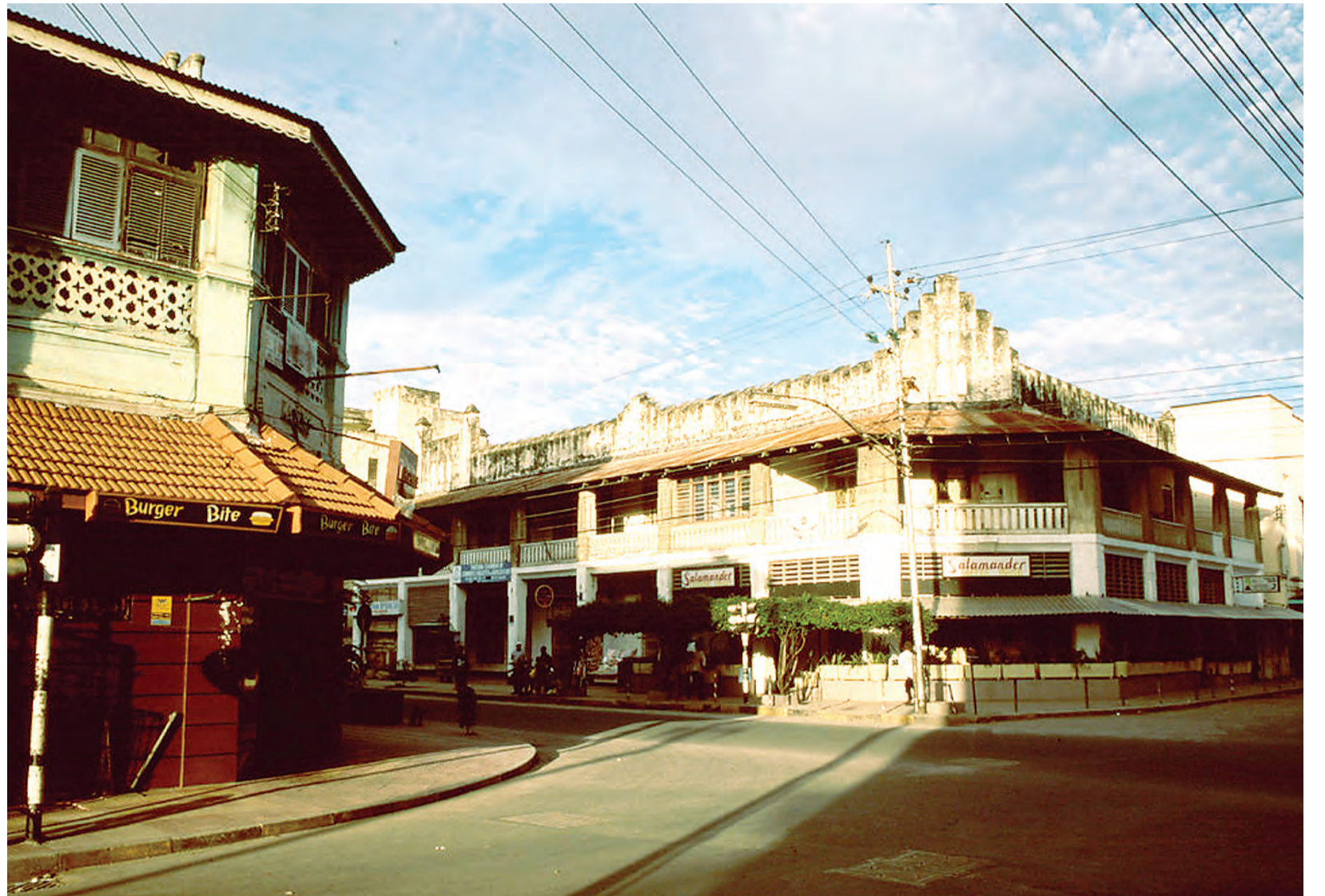
A Dar es Salaam gem, the old German building that once housed the popular Salamander Cafe, which was demolished along with much else historic value in the city centre. Many such structures have often been declared unfit for human habitation and often sold off to dubious developers. Can we be sure therefore, that what little is left in the conservation category is now soundly safeguarded.
