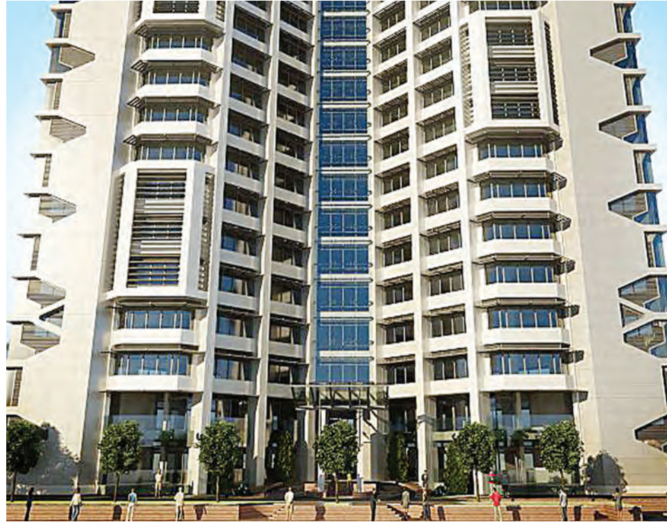
Proposed headquarters of the Pan African Postal Union (PAPU) building in the city of Arusha
