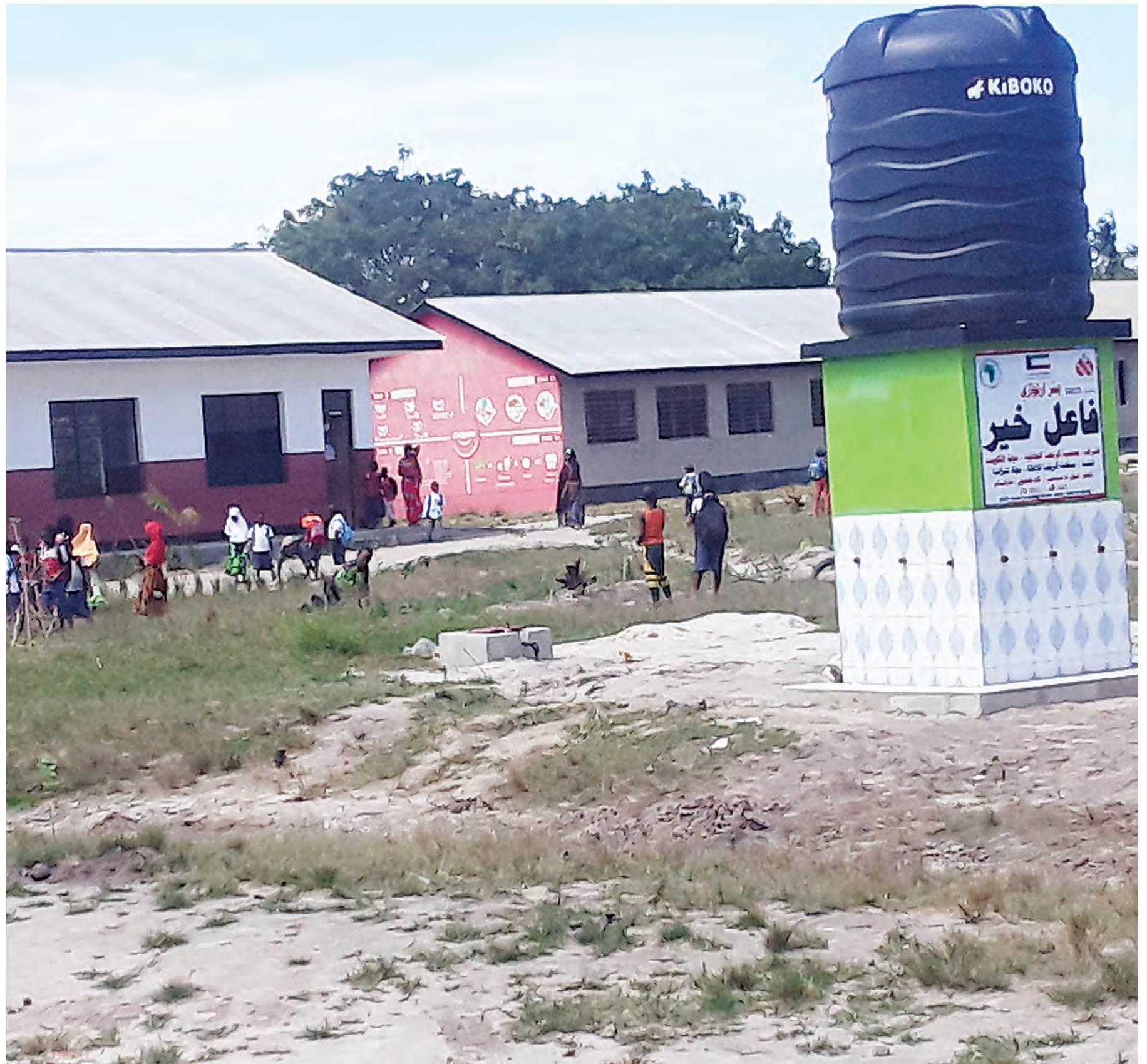
Water tanks near a water well at Kivule Annex Primary School which was constructed by the government of Tanzania in support of the African Relief Organisation Tanzania in collaboration with the Kuit-Rahma International Society. Photos: Correspondent Daniel Semberya
