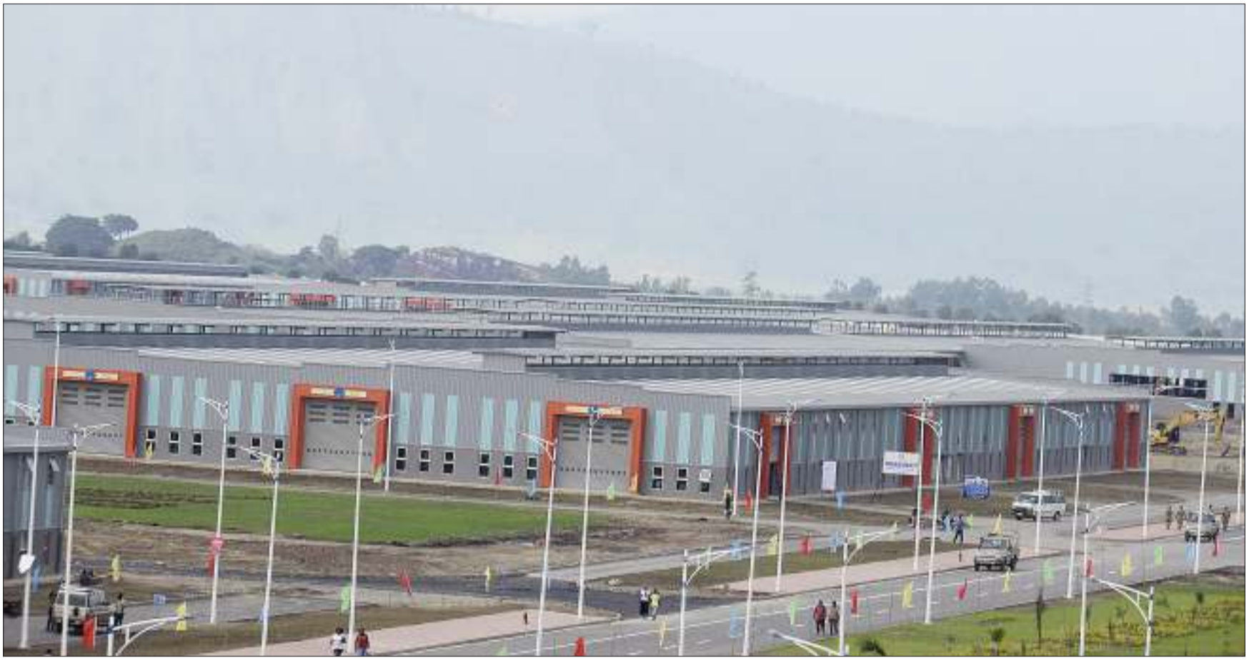
Hawassa Industrial Park, which the Ethiopian government considers as its flagship industrial park in its ambition to transform the country as the manufacturing hub of the African continent by 2025, was built by China's Civil Engineering Construction Corporation and completed in 2016 after just nine months of construction. File photo
