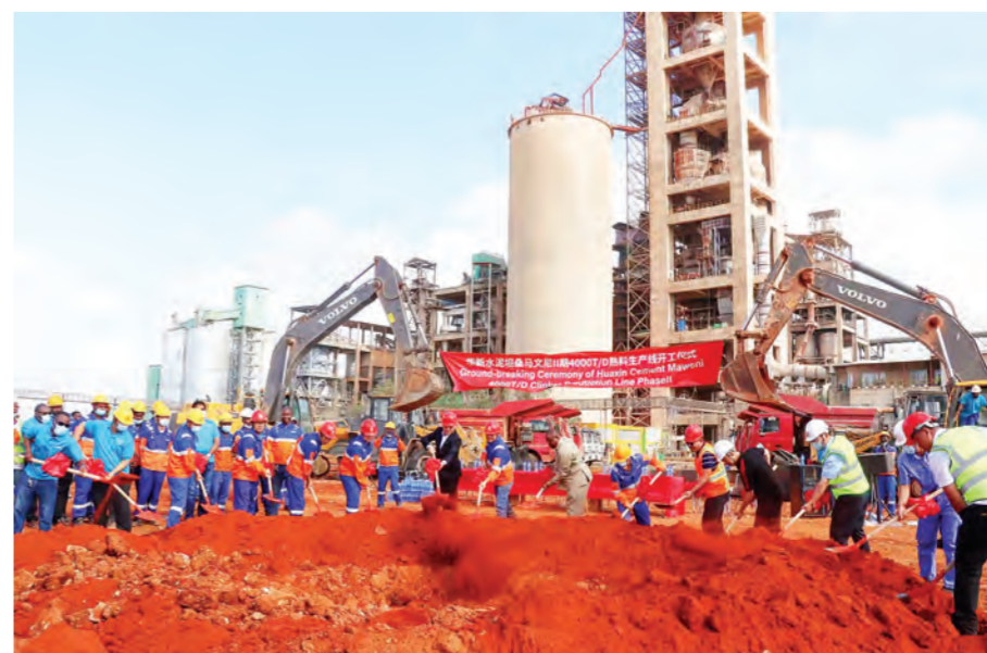
The groundbreaking launch of Phase II of the Huaxin Maweni 4000T/D clinker production line as held at Maweni in Tanga District, Tanga Region, on July 26, 2022. File Photo
