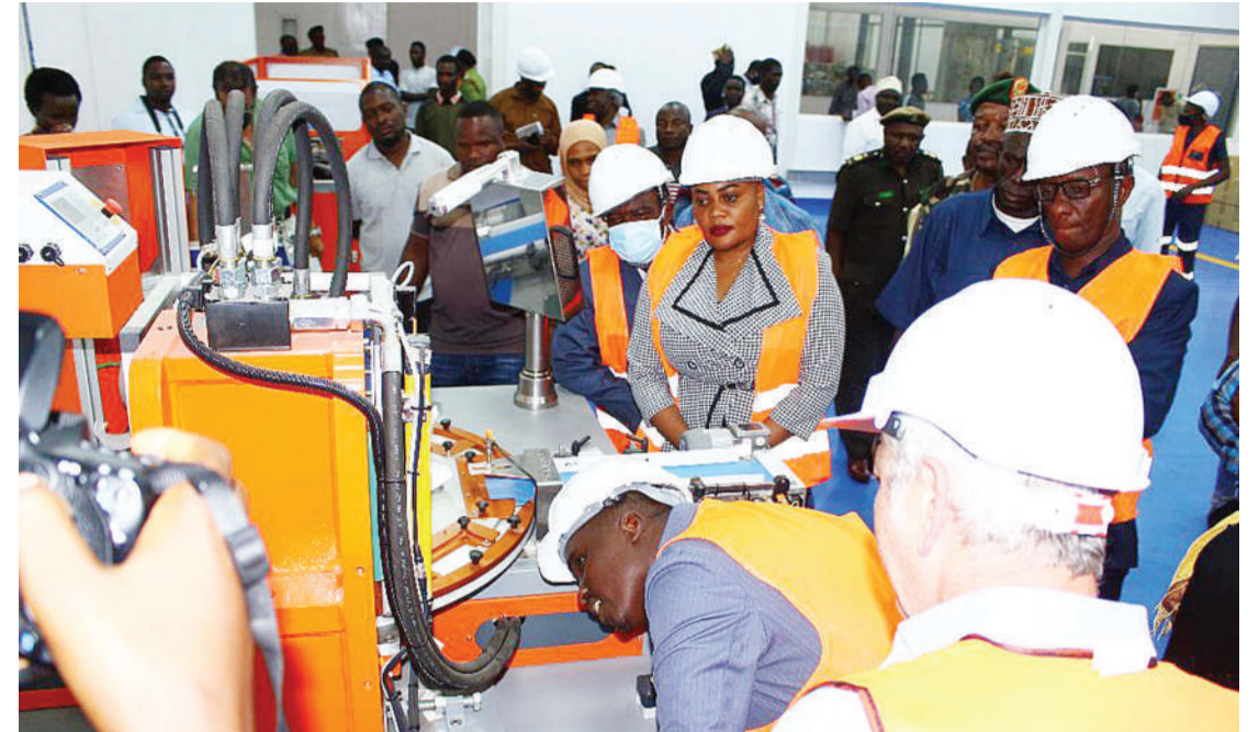
Minerals Minister Dotto Biteko takes a close look at modern mining equipment installed at Geita Gold Refinery when he visited the factory last week. Photo: Guardian Correspondent.
