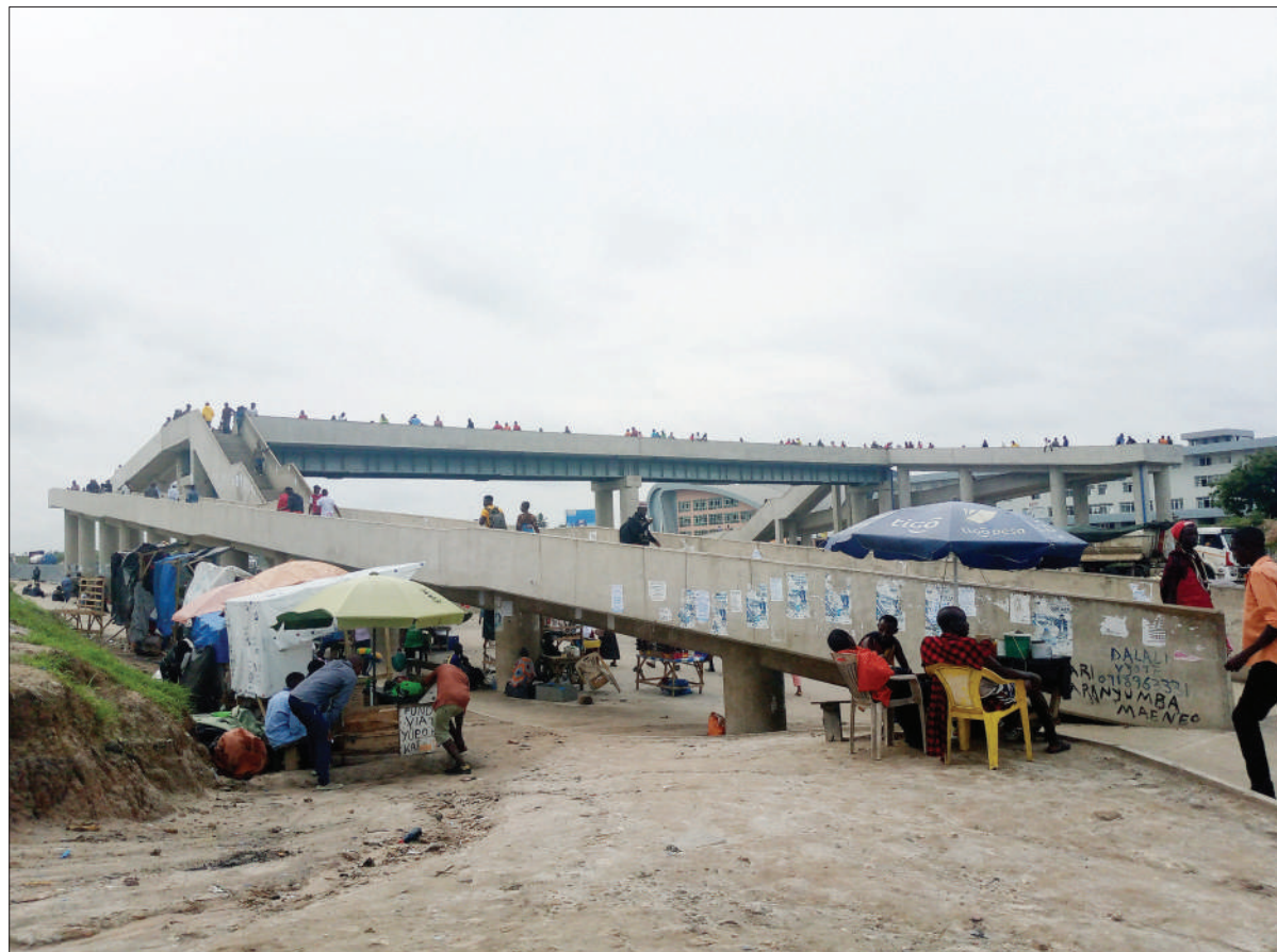
Pedestrians bridge at Mbezi Luis in Dar es Salaam is almost completed but some residents do not use it and preferred to cross Morogoro road by penetrating through the fence as captured yesterday. Photo: Correspondent Sabato Kasika
