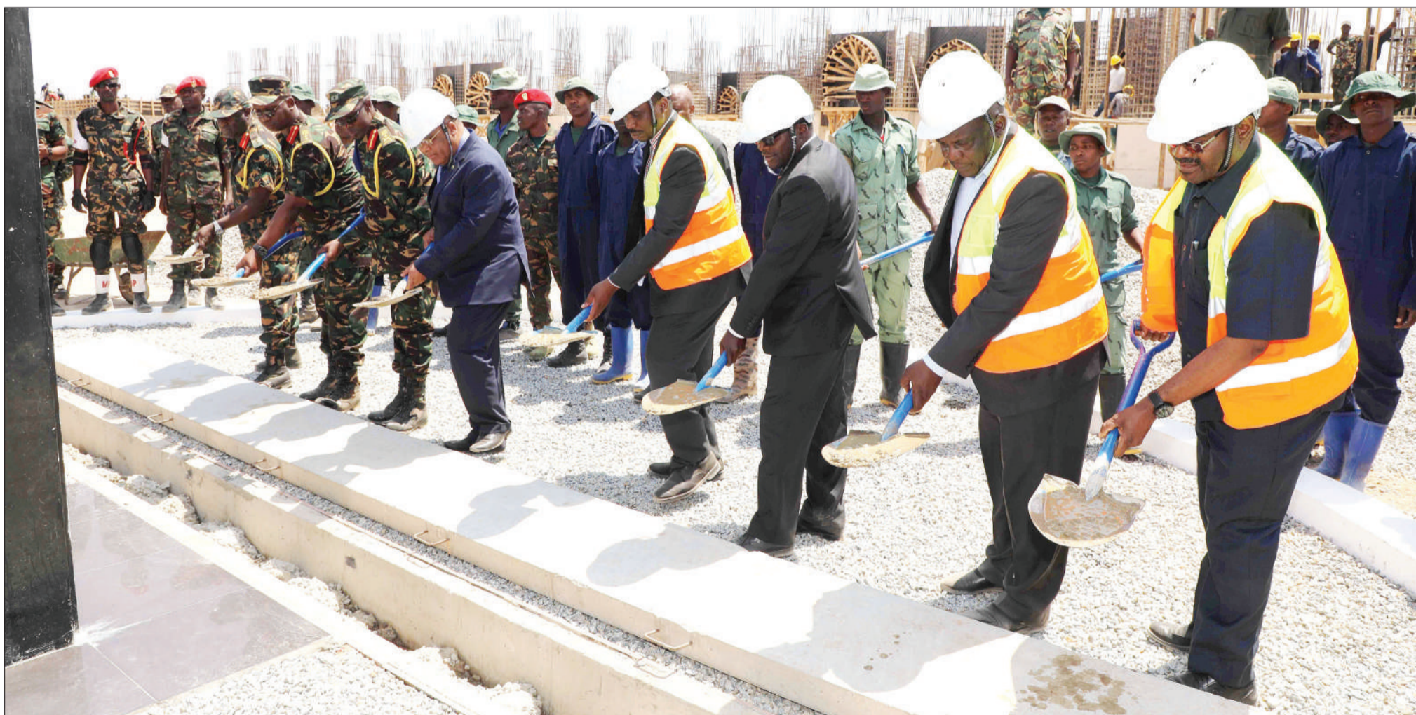
Chief Secretary John Kijazi (5th-R) leads ministerial permanent secretaries and their deputies at Chamwino in Dodoma Region yesterday in sprinkling soil on the foundation of a building undergoing construction at the Chamwino State House compound. They were on a routine tour. Photo: State House.
