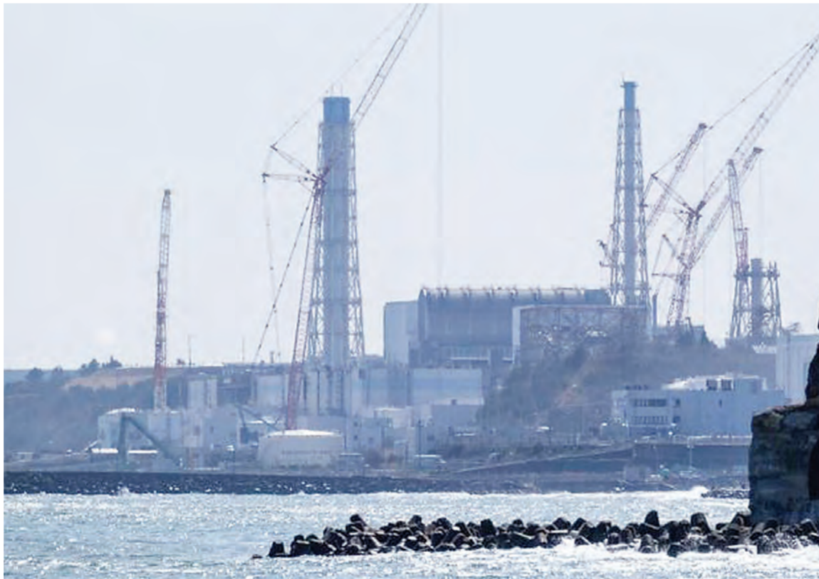
Tokyo Electric Power Company Holdings (TEPCO) Fukushima Daiichi nuclear power plant is seen from the coast of Futaba town in Fukushima prefecture.
