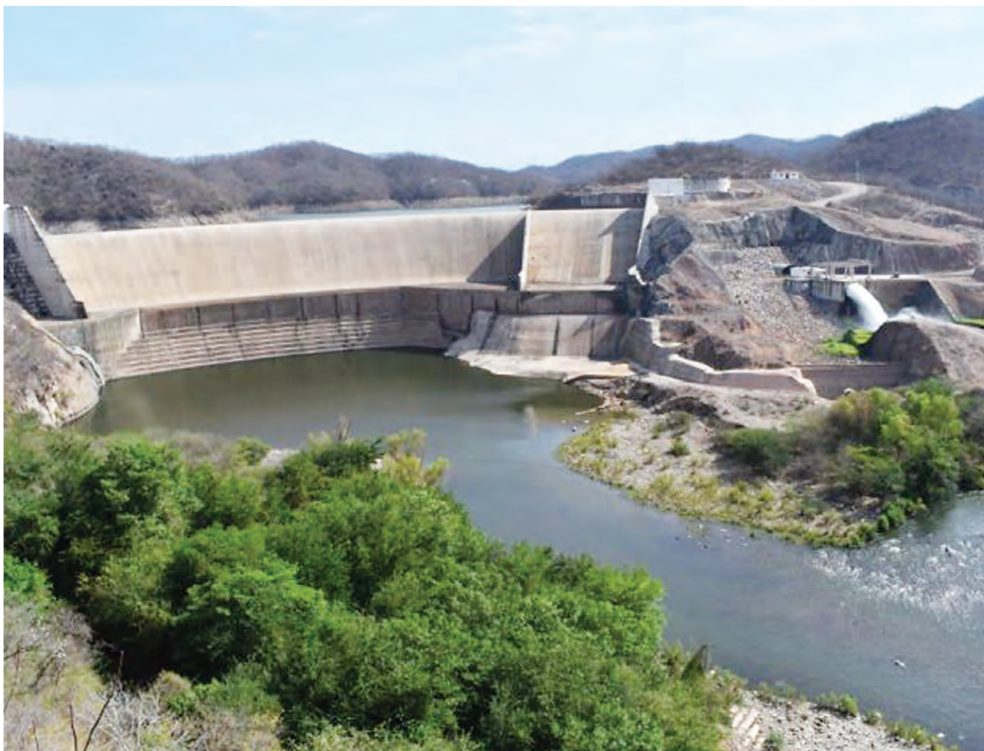
With a storage capacity of 580 million cubic meters and an irrigation target of 22,500 hectares, the Picachos dam in the state of Sinaloa, in northwestern Mexico, will also generate 15 megawatts of electricity. CREDIT: Conagua
