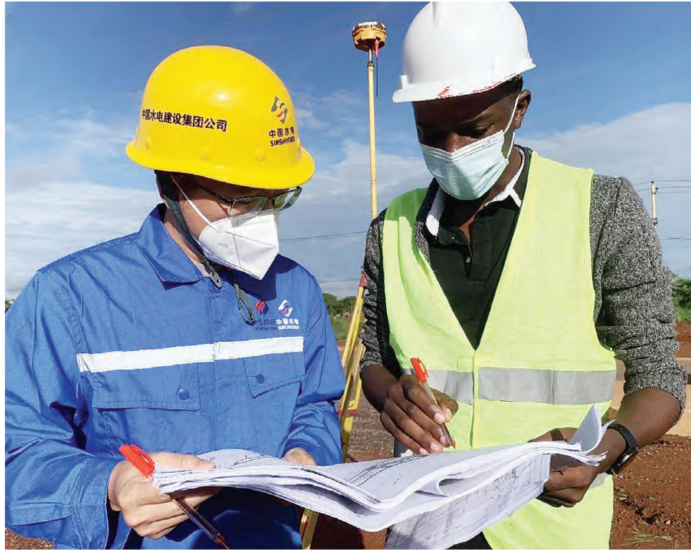
Chinese and Ugandan engineers discuss construction plans at the construction site of the Karuma Hydro Power Plant in Uganda, which is built by Power Construction Corporation of China. (Photo provided by Power Construction Corporation of China)
