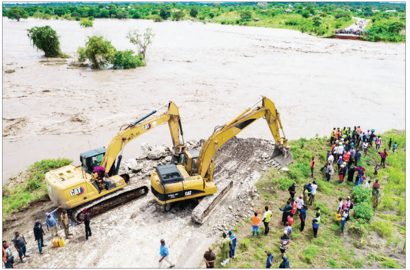
Cyclone Hidaya has come and gone, leaving behind a trail of unprecedented destruction with grave economic and other consequences. This is part of the heart-rending evidence: what was until only two or so days ago a rock-solid Nangurukuru stretch of the strategic all-weather tarmac highway linking Dar es Salaam city and Mtwara municipality via Lindi municipality, as caught yesterday. But contractors have already swung into action and are working around the clock, with the government promising completion of the rehabilitation of the infrastructure - again, within a day or two. Photo: Works ministry
