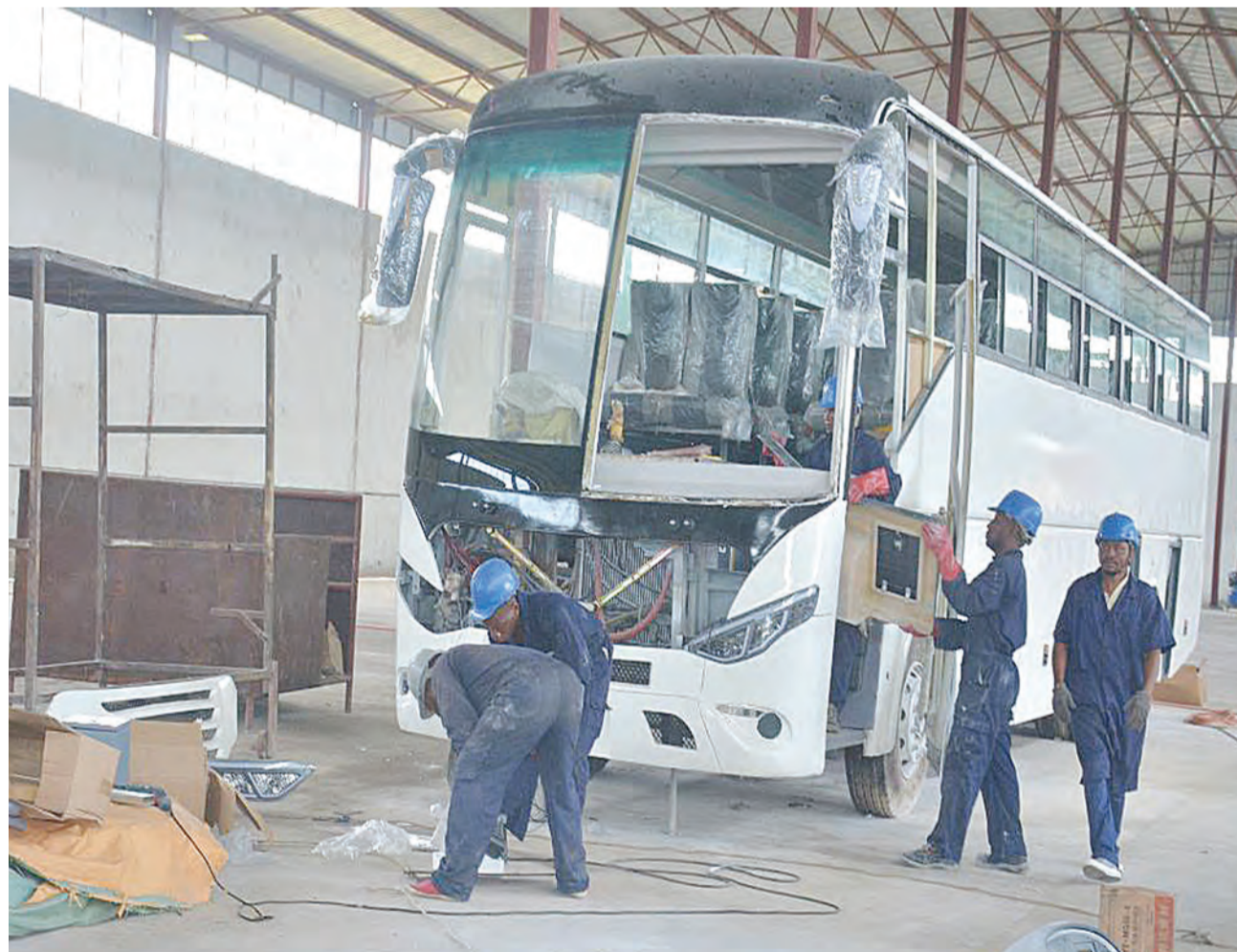
BM Assembling Plant employees at work at their Kibaha factory premises. Photo courtesy of NIT.
