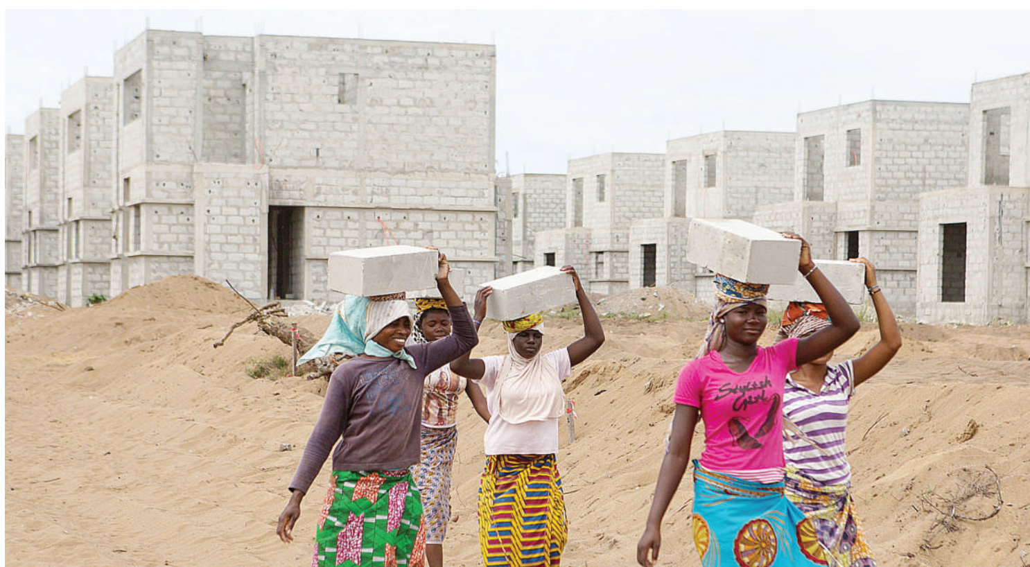
Women working at a commercial property construction site in Lagos.
