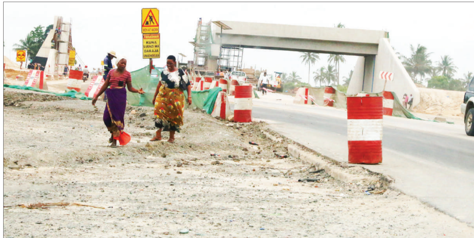
This is the current look - as captured yesterday - of the overhead bridge at Kibamba in suburban Dar es Salaam meant to enable pedestrians to cross the envisaged six-lane stretch of Morogoro Road with enhanced assurance of safety. The all-important road is undergoing massive expansion, chiefly as a decongestion measure. Photo: Selemani Mpochi
