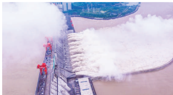
The Three Gorges project opens 11 deep spillway holes to discharge floodwater.
