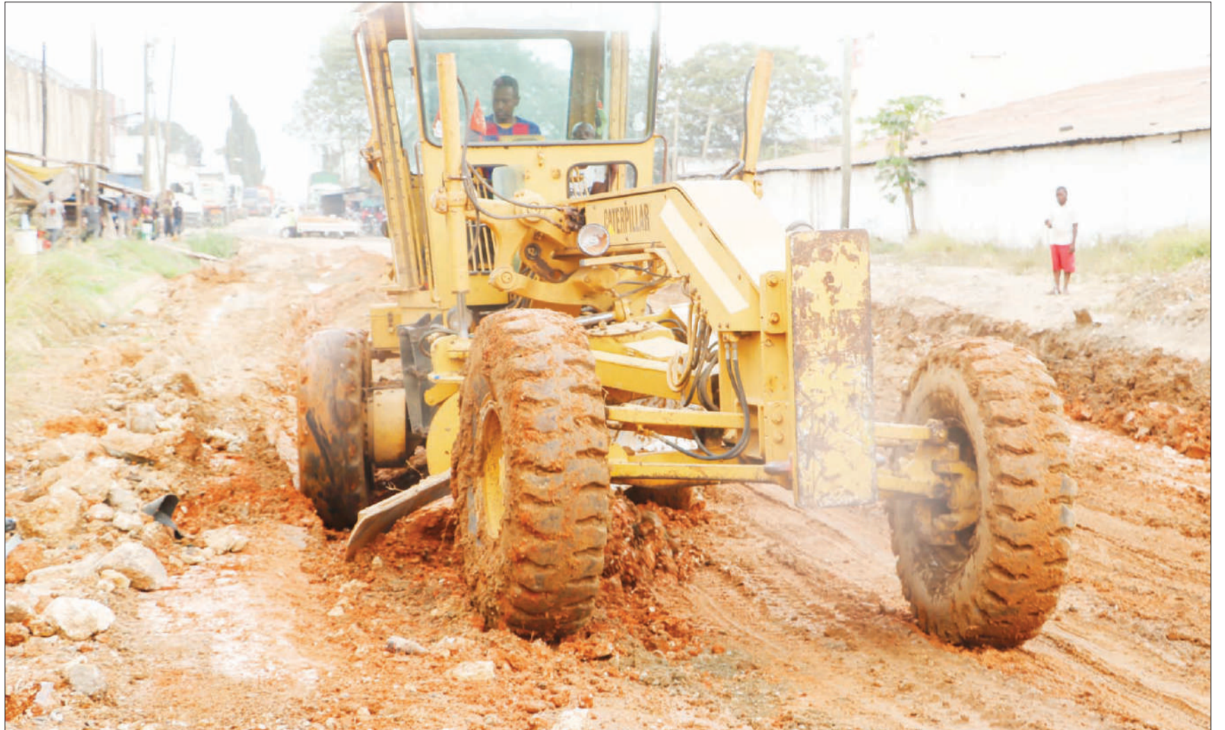
A road grader employees at work along Mwakangale road in Temeke District, Dar es Salaam which had been destroyed during the recent rainy season. Photo: Correspondent Jumanne Juma
