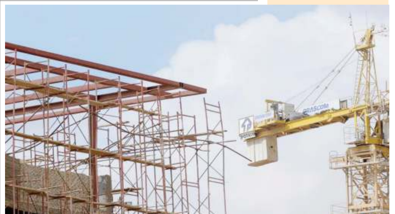
Orascom Construction's site in Cairo.
