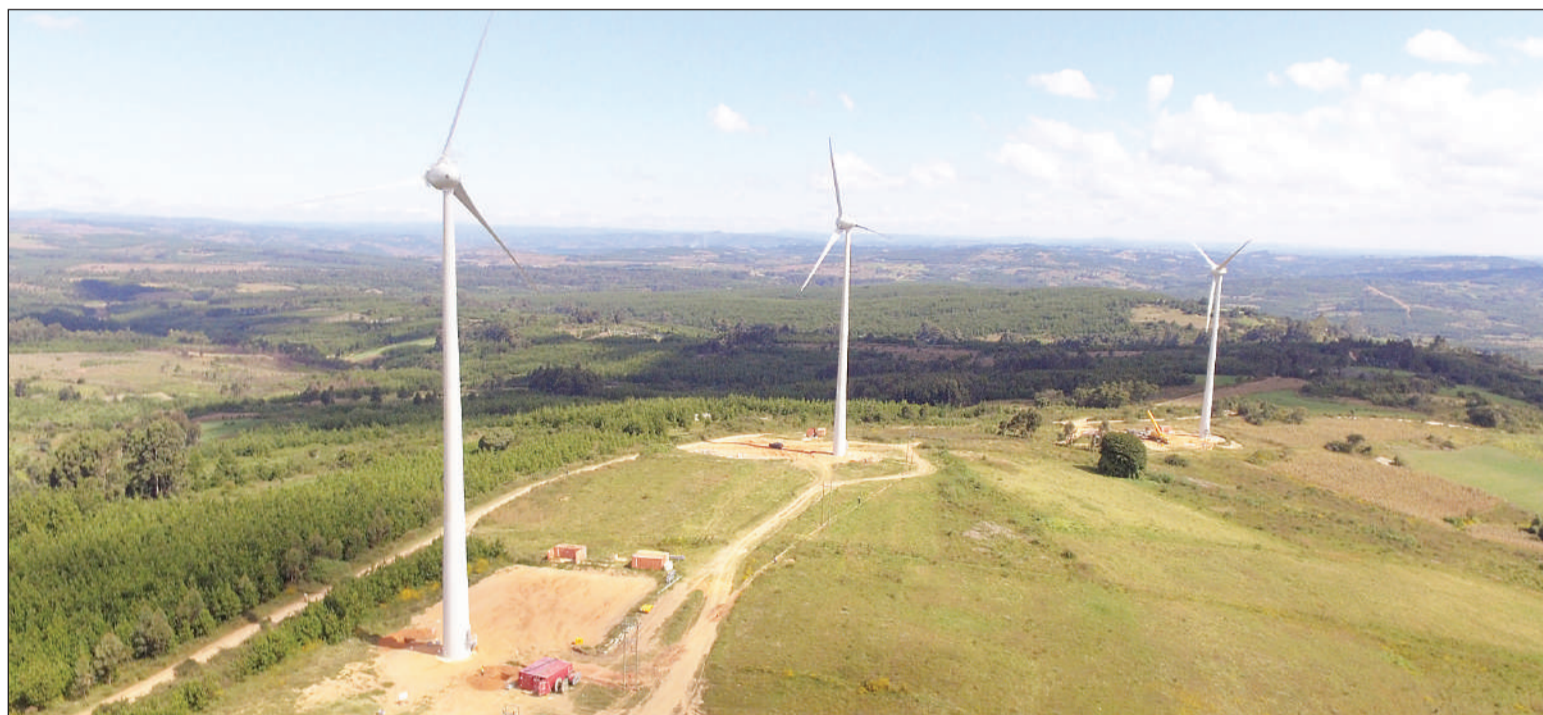
An aerial view of Mwenga Power plant's three turbines of which one is already on test trials.
