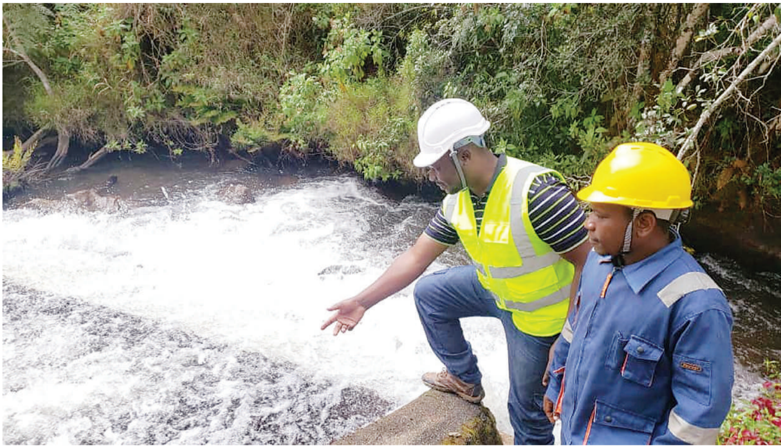
The Luponde Hydro and Rural Electrification Power Project (LHREPP) project manager Eng. Maxwell Mugombe (L) and Msafiri Kalinga, assistant power plant operator look at the operation of the pelton turbine for the 0.9 MW LHREPP project in Njombe District, Njombe Region.
