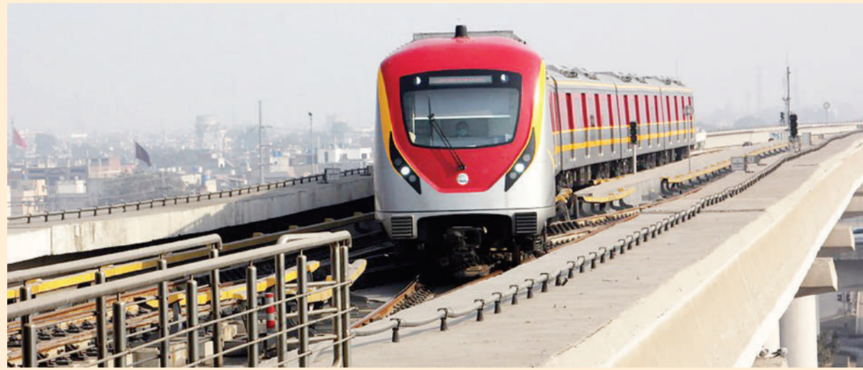
An Orange Line metro train pulls into the terminal station in Lahore, Pakistan, Dec. 29, 2021. Officially open to traffic on Oct. 25, 2020, the eco-friendly Orange Line metro train is an early project under the China-Pakistan Economic Corridor (CPEC), a flagship project of the China-proposed Belt and Road Initiative. Xinhua
