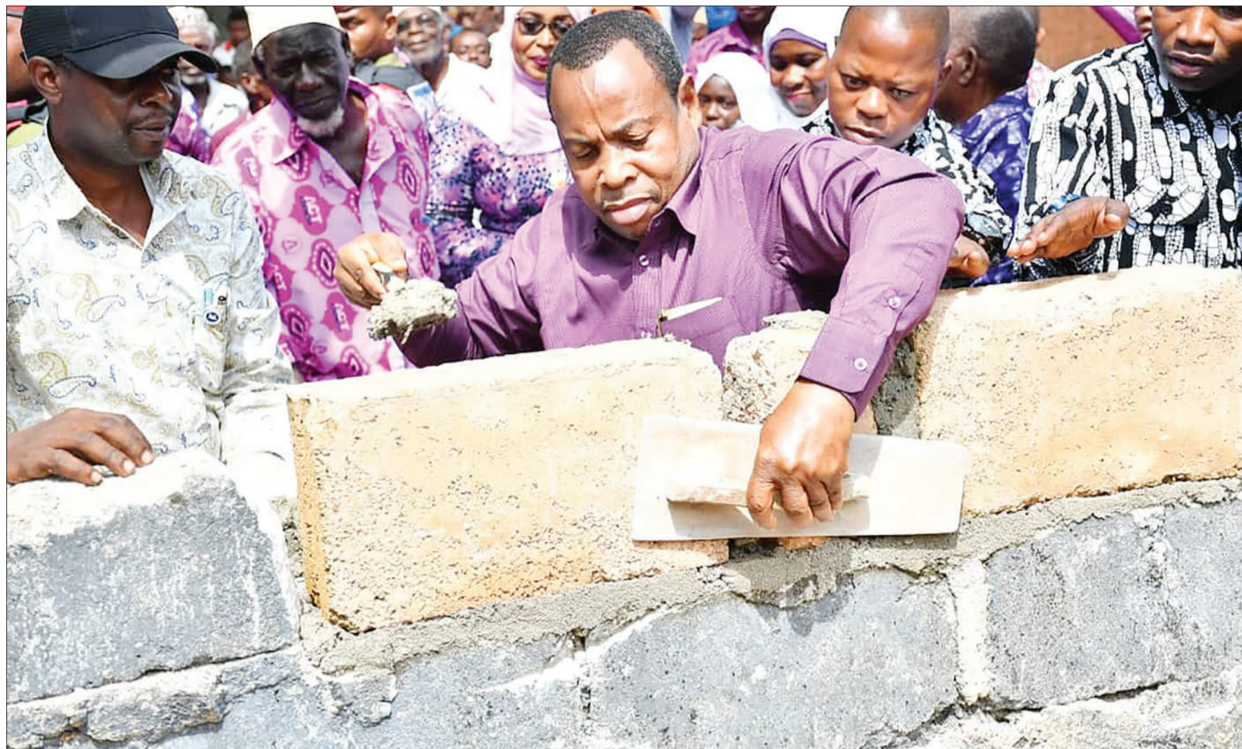
Zanzibar First Vice President Othman Masoud Othman (3rd-L), who is also Vice Chairman (Zanzibar) of the opposition ACT-Wazalendo, lends a hand in construction work on the party's office at Shakani Makunduchi in South Unguja yesterday. Photo: Rahma Suleiman
