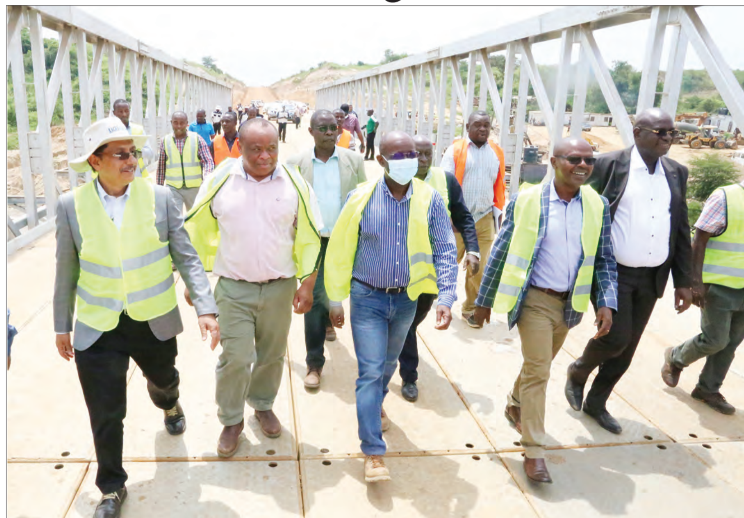
Works and Transport minister Prof Makame Mbarawa (3rd L) inspects Kitengule bridge connecting Misenyi and Karagwe districts in Kagera region shortly after visiting the Kagera Sugar factory yesterday. Left is KSL board chairman Seif Ali Seif and (2nd R) is Misenyi District Commissioner Col. Denis Mwila. Photo: Selemani Mpochi
