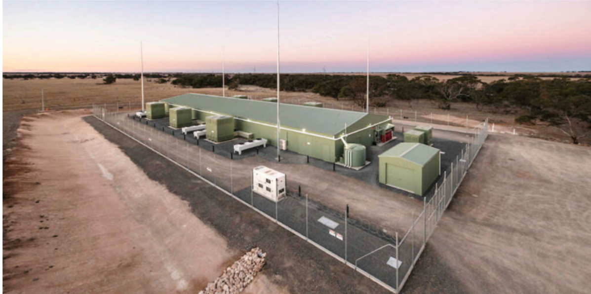
The first BESS in Australia with 'virtual synchronous machine' capabilities of delivering inertia to the grid PHOTO/HITACHI
