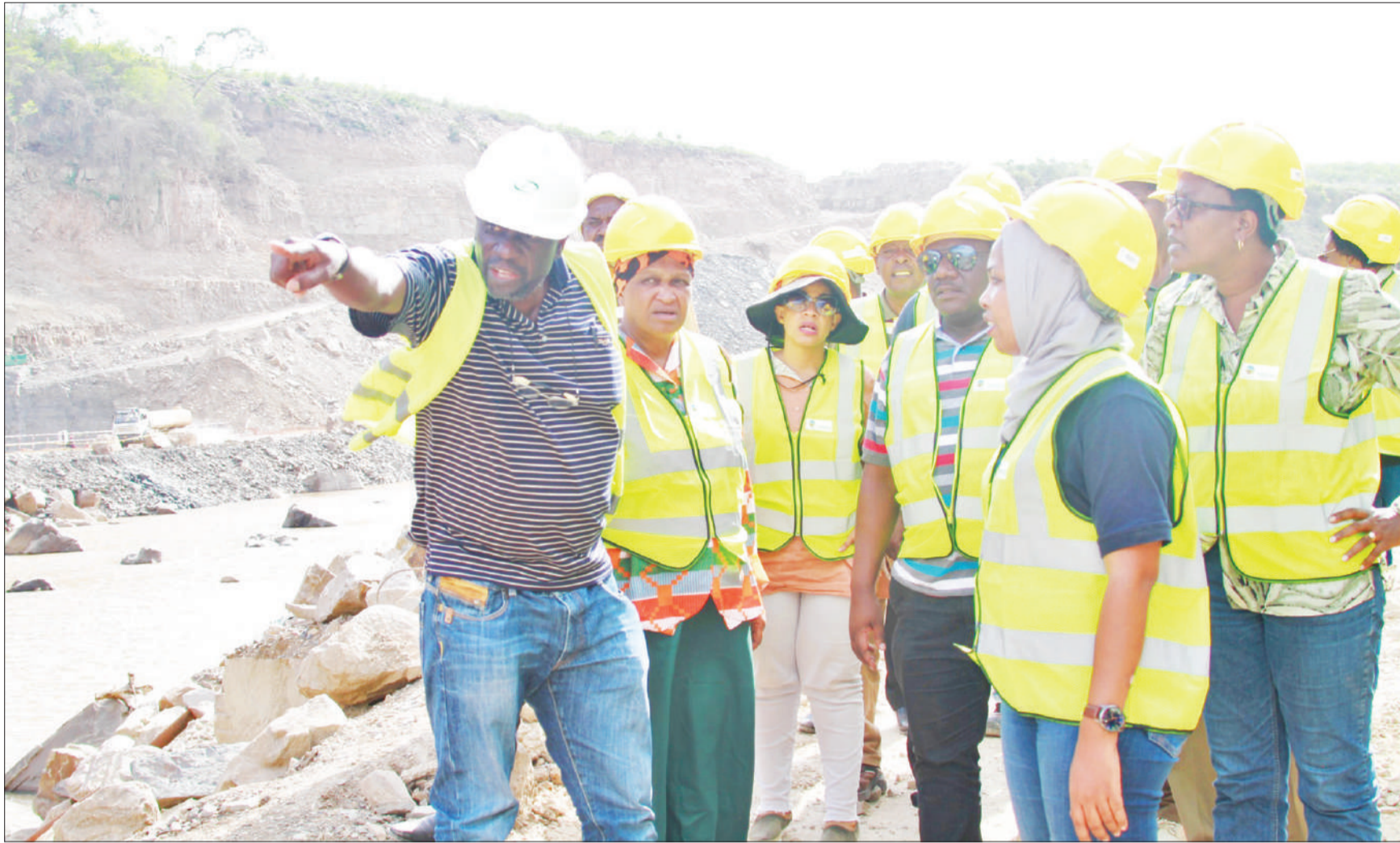
Dr Majige Mabulla (L), head of the occupational health and safety unit of the Tanzania Electric Supply Company Limited (Tanesco), briefs National Environment Management Council (NEMC) board members during their one-day visit to Julius Nyerere Hydropower Project (JNHPP) site in Rufiji District, Coast Region, at the weekend. Second left is the board's chairperson, Prof Esnat Chaggu. Photo: Guardian Correspondent
