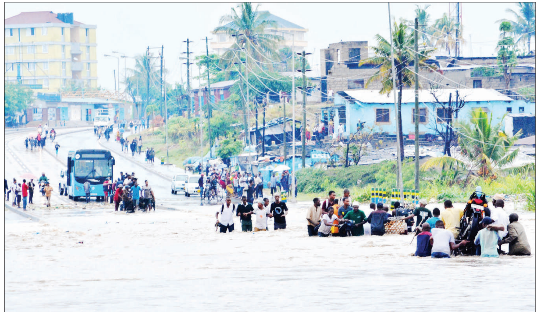
A scene captured yesterday afternoon at the Kinondoni Mkwajuni section of Dar es Salaam's Kawawa Road - under floodwaters and hardly passable a few hours after a day-long downpour pounded the city. Photo: Correspondent Miraji Msala
