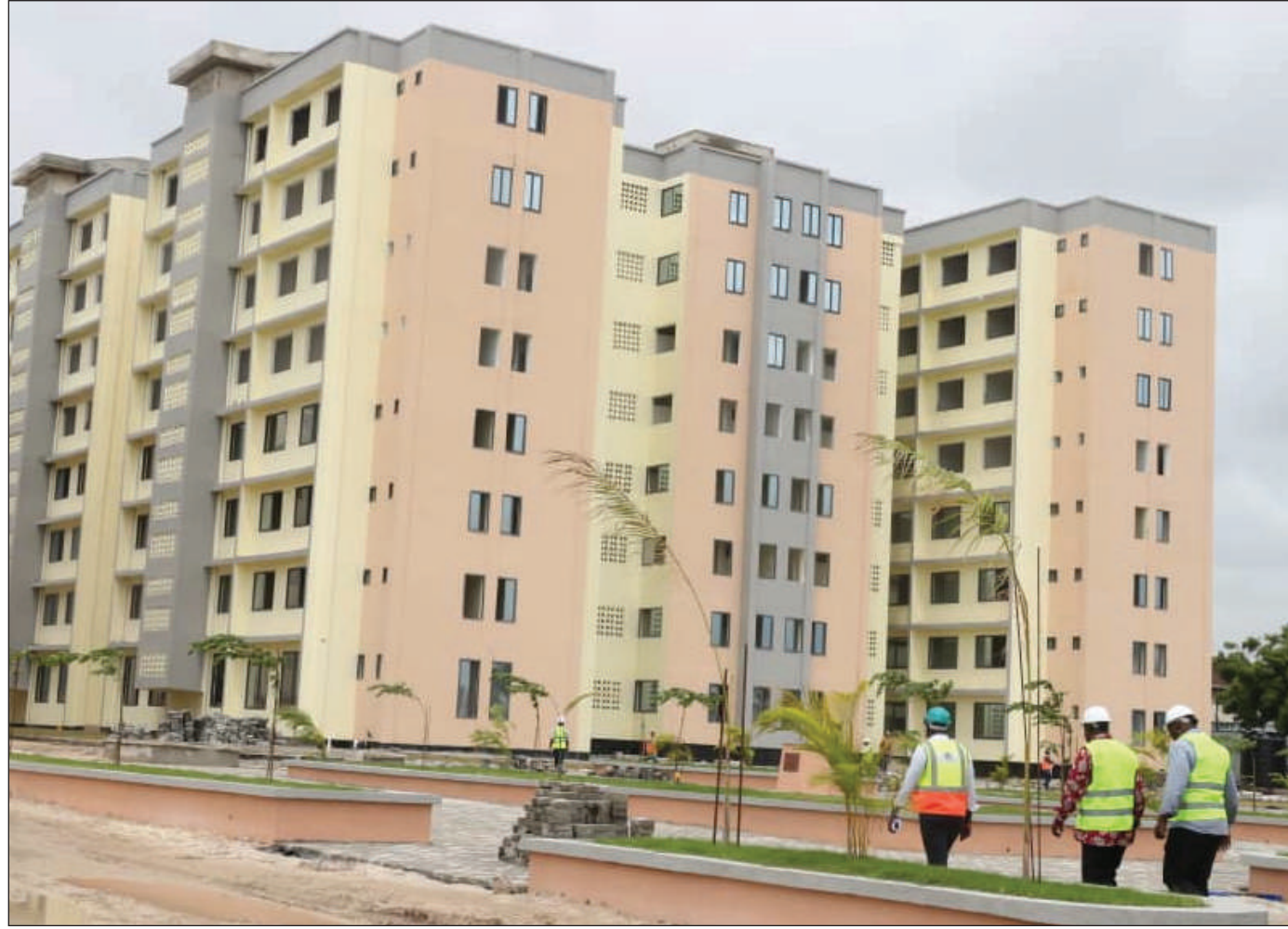
New Magomeni apartment blocks in final stages of construction.
