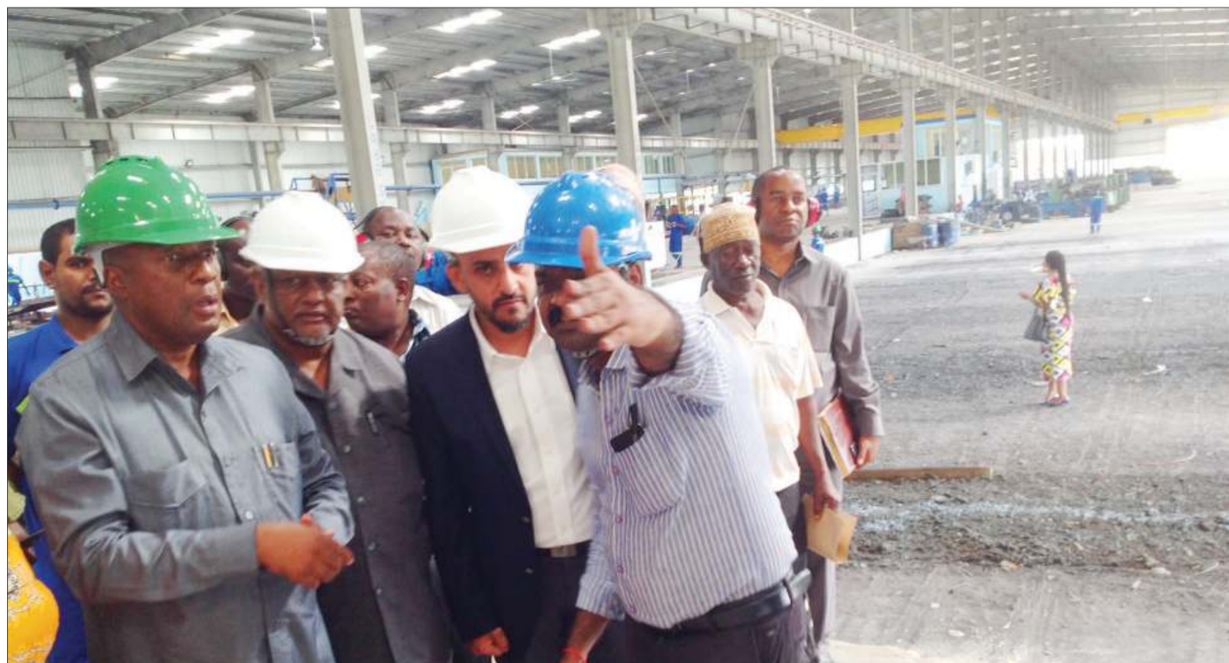
A Lake Group official explains to Coast regional commissioner Evarist Ndikilo (L) at Kibaha yesterday after he had laid foundation stones for the firm's factories meant to make gas cylinders, iron bars and water pipes. Photo: Guardian Correspondent
