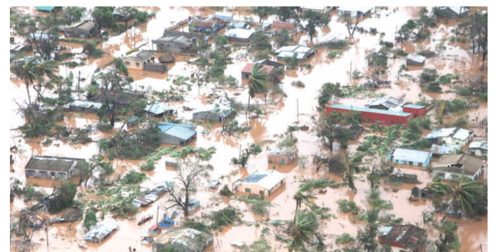
Flooding from Cyclone Idai and Cyclone Kenneth affected 2.2 million people in Mozambique. File photo
