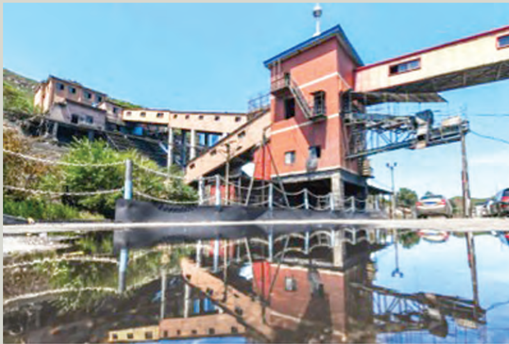
Photo shows a conveyor belt and a coal warehouse at the Datai coal mine, Beijing.
