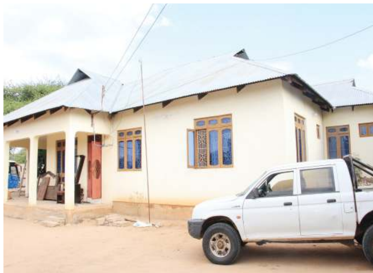
Manyoni lawmaker, Yahaya Masare's family house at Uzunguni street in Dodoma city which TRA mistakenly rated as a 100,000/- property tax facility. Photo: courtesy of Ministry of Finance.
