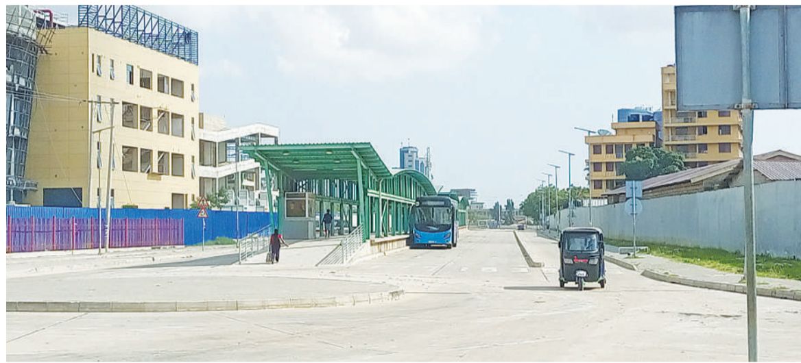
A Rapid Transit bus station in Dar es Salaam. Photo: Francis Kajubi.
