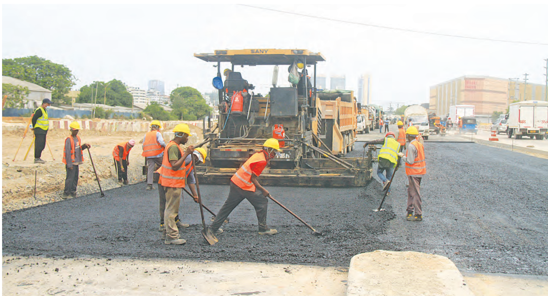
Construction workers lay tarmac along Nyerere Road at Darajani Chang'ombe area in Dar es Salaam, yesterday. Photo: Correspondent Jumanne Juma
