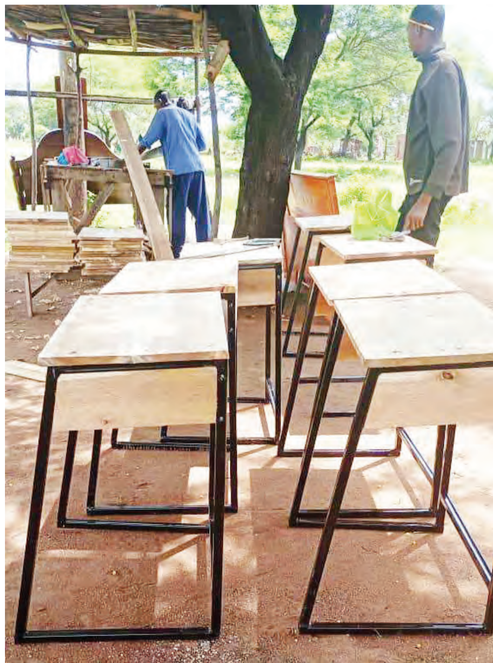
Carpenters make desks for pupils set to begin Form One at Muhoji Secondary School, Bugwema Ward in Musoma Rural Constituency, Mara Region, at the weekend. Photo: Correspondent
